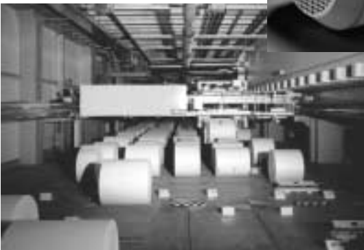
Motors and drives in a paper mill (Copyright ABB)
