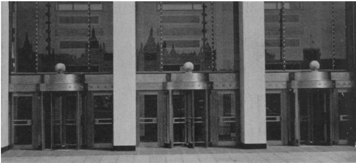
Already a well-known London landmark, the Shell Centre at South Bank, like many other prestige buildings, has nickel silver entrance doors
