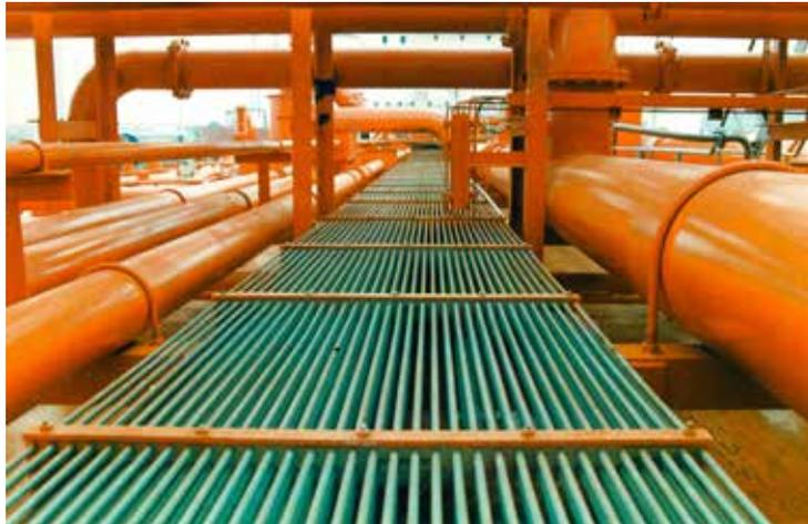
*Figure 1 - 90/10 copper-nickel piping on a marine chemical tanker
