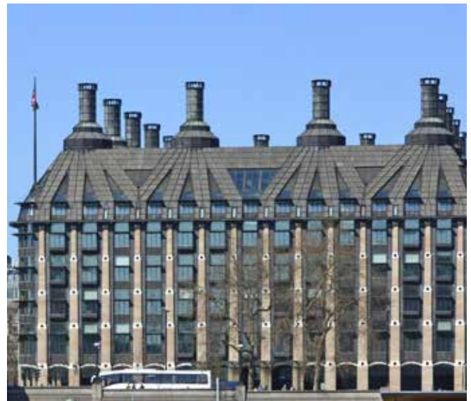
Figure 4 – Nickel aluminium bronze roof, Portcullis House
