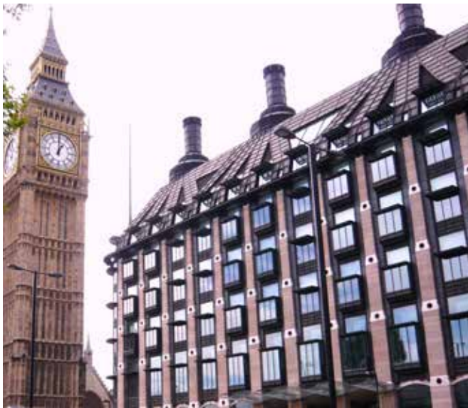
Figure 3 – Nickel aluminium bronze window frames, Portcullis House
