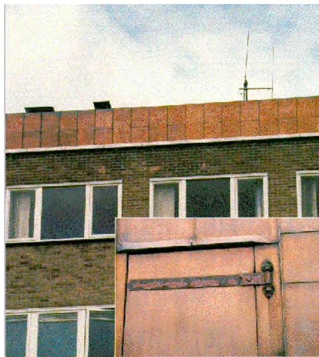
Enfield Rolling Mills in North London
